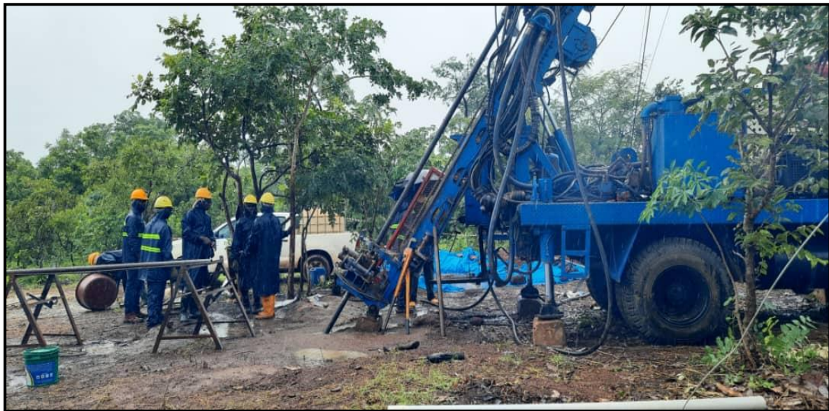
Figure 12. Core drilling activities in the field.
